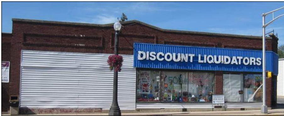
Existing Underutilized Building
